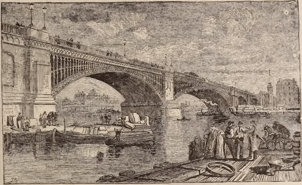
CHESTNUT STREET BRIDGE.
